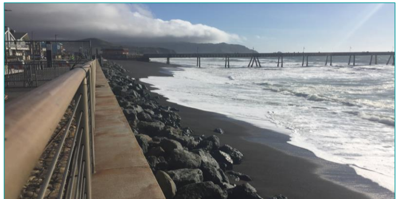
Beach Boulevard Seawall, looking south.
