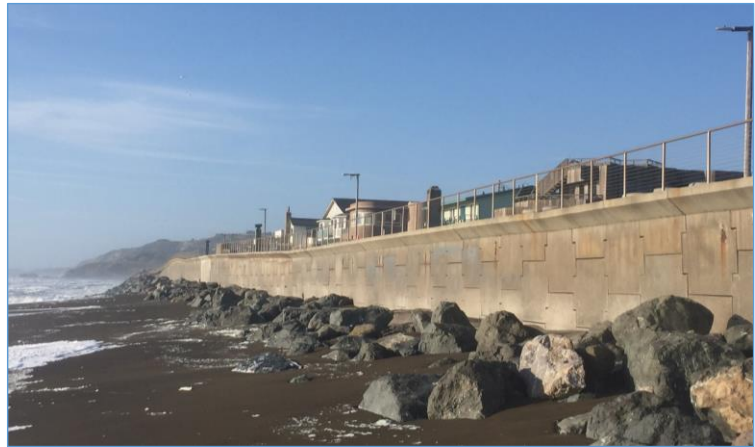
Beach Boulevard seawall from the beach, looking north.
