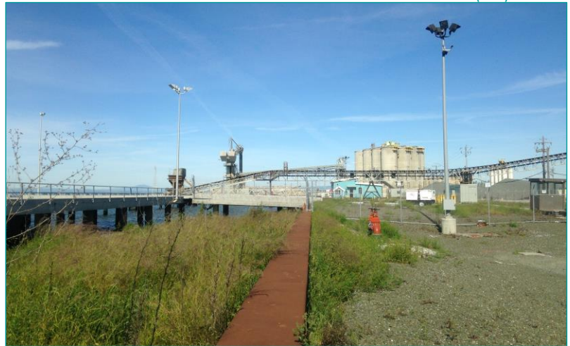
New seawall at the Port with tenant facilities and new wharf (left).
