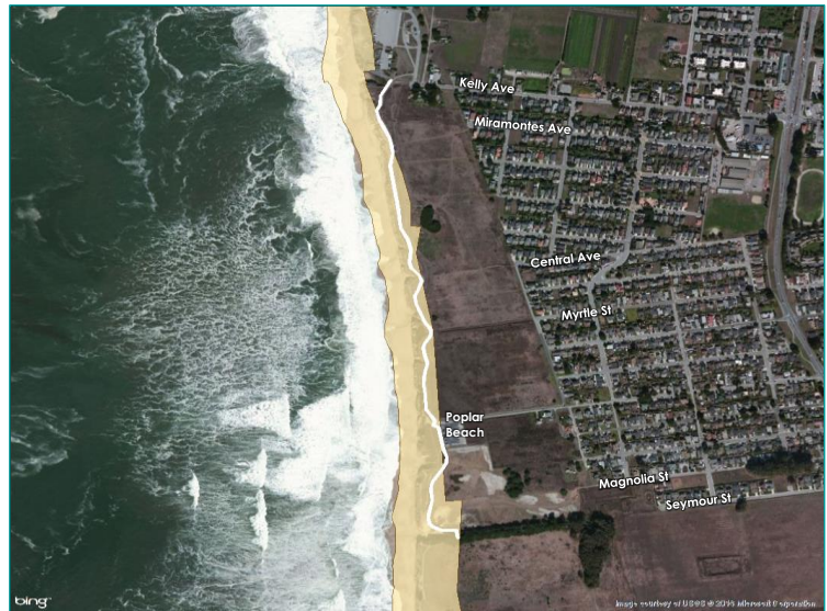
Asset is nearly entirely within the 2100 erosion zone.
